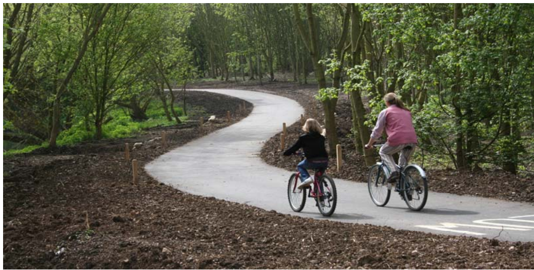
Landscaping delivering a mix of woodland, pathways, cycleways and wildlife habitat
